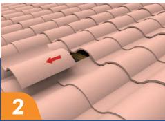
Remove the tile where you are installing the hook by gently pulling and pushing the tile.
