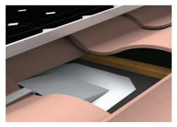
Apply sealant to the bottom portion of the flashing. Attach to the roof with roofing nails; apply sealant.
