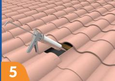
Backfill both pilot holes with sealant.
