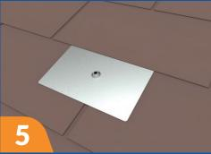
Insert the Chiko Solar flashing under the shingle as far as possible. This will ensure there is no water infiltration
